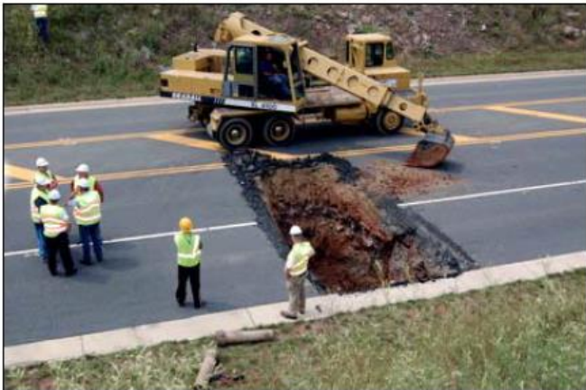
Approximately one year later, the sinkhole reopened at the same location. The sinkhole is approximately 20 feet in diameter and 15 to 18 feet in depth. (photograph date: June 29, 2006; source: Leesburg Today)
