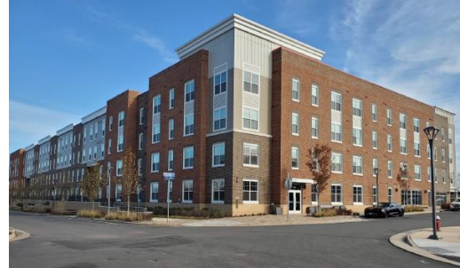
Heronview Apartments (96 units, Kincora, VA)
